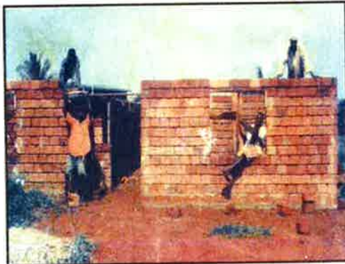
INTERLOCKING BLOCK HOUSE UNDER CONSTRUCTION
