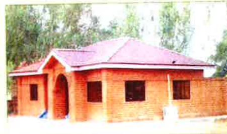
BUILDING WITH STABILISED BRICKS
