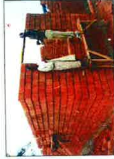
INTERLOCKING HOUSE UNDER CONSTRUCTION
