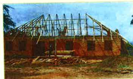
A HOUSE UNDER CONSTRUCTION USING THE CINVA RAM BRICK SYSTEM
