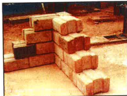
BOLYN INTERLOCKING BRICK LAYING METHOD
