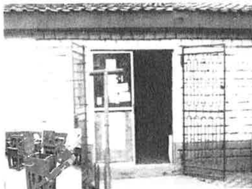
BOLYN CONSTRUCTIONS CO. LTD HEAD OFFICE - BUILT USING NO MORTAR INTERLOCKING BLOCK + CONCRETE ROOF
