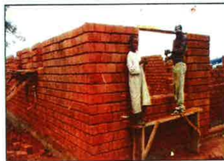
INTERLOCKING HOUSE UNDER CONSTRUCTION
