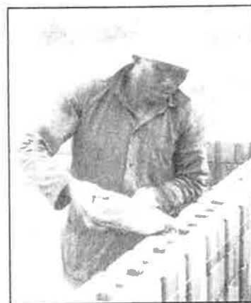
Pouring Cement Grout into Brick Holes to form Mortar Joints
